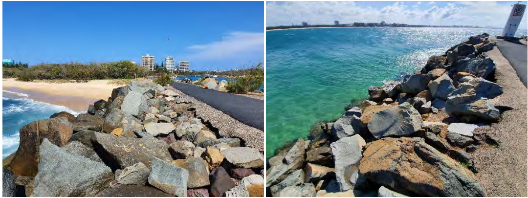
Figure 3.1 Existing Mooloolaba breakwater. Left: looking southeast along the seaward side of the breakwater. Right: Looking northwest along the leeward side of the breakwater. Signs of rock slumping and undermining of the concrete blinding layer under the footpath observed. Wide rock grading also observed.
