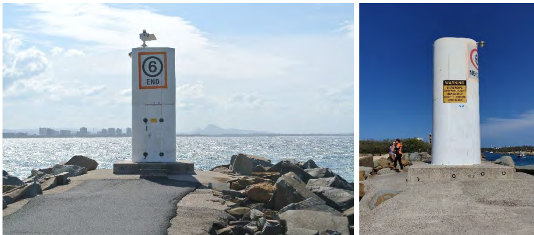
Figure 3.4 Existing navigation beacon. Left: landward perspective towards the northwest. Right: seaward perspective looking towards the southeast.
