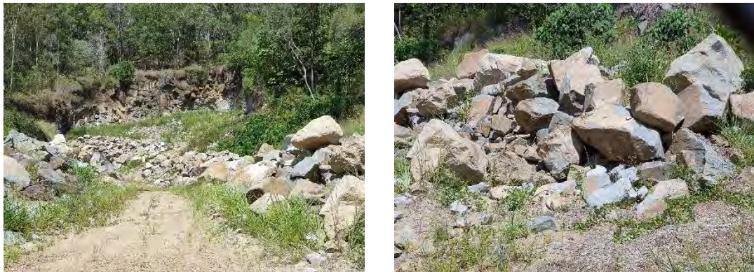
Figure 2.1 View into Kuluin Quarry and rock armour stockpiles from Commercial Road, Kuluin. Larger pictured armour is estimated to have a median diameter ( D_{50} ) of about 1.2 m at 15 March 2019.
