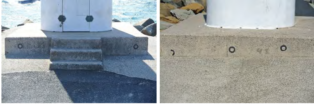
Figure 3.5 Base of existing navigation beacon and pad footing slab. Left: landward perspective towards the northwest. Right: seaward perspective looking towards the southeast.
