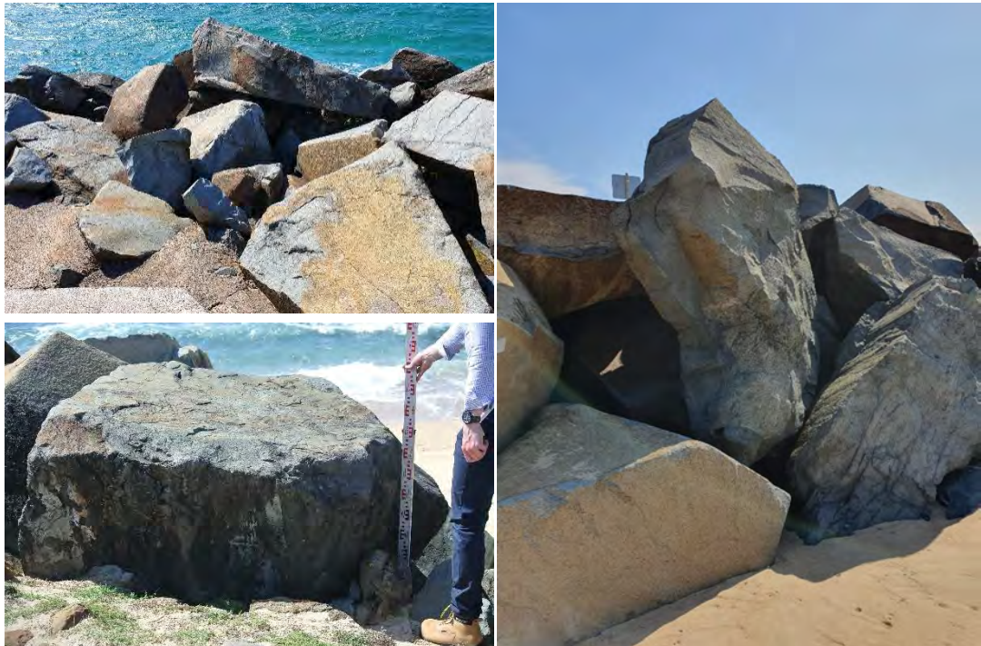
Figure 3.2 Primary rock armour along the existing eastern Mooloolaba breakwater. Considerable rock aspect ratio deficiencies noted in some instances. Right: aspect ratio approximated to be L/E = 2.5 \text{ m}/0.5 \text{ m} = 5 .
