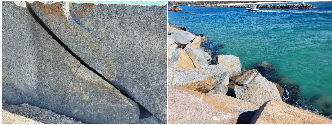
Figure 3.3 Left: cracking of rock armour on the leeward crest of the existing breakwater. Rock believed to have been sourced from the Kuluin Quarry. Right: potential signs of rock instability on the leeward side of the existing breakwater.
