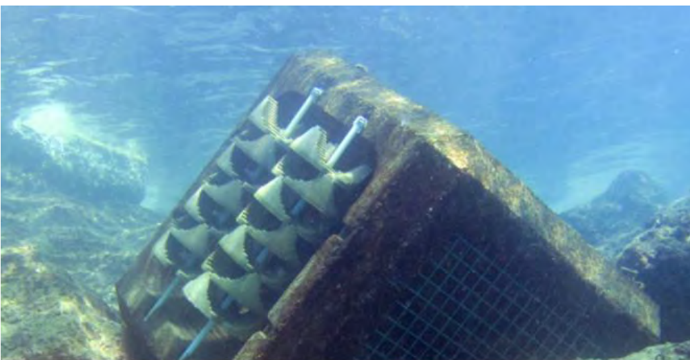
Figure 5 Insitu EConcrete ECO Armour Block with add-on elements attached to the block faces
