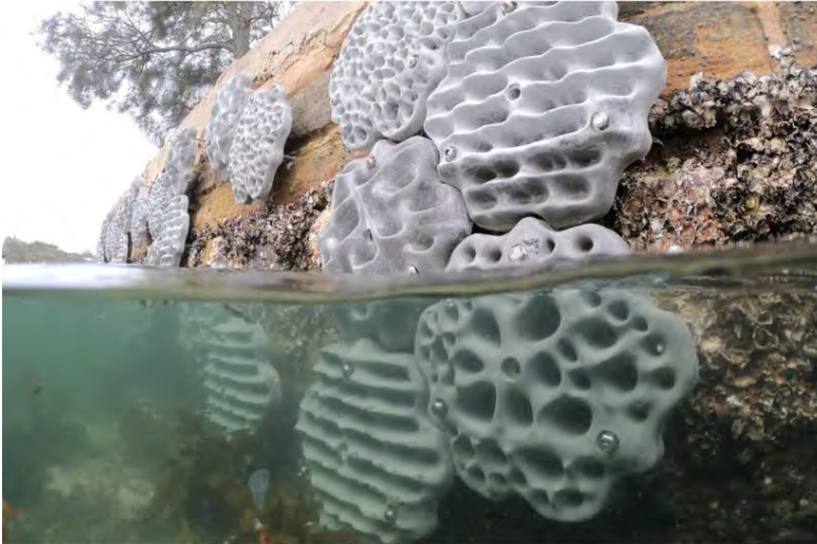
Figure 2 Living Seawalls installation in Sydney (Source: Reef Design Lab)
