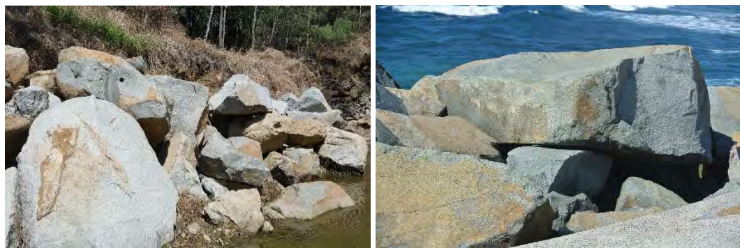
Figure 4.4 (a) Stockpiled Kuluin Quarry Rock and (b) Armour rock on the crest of the Mooloolaba Breakwater (seaward side)
