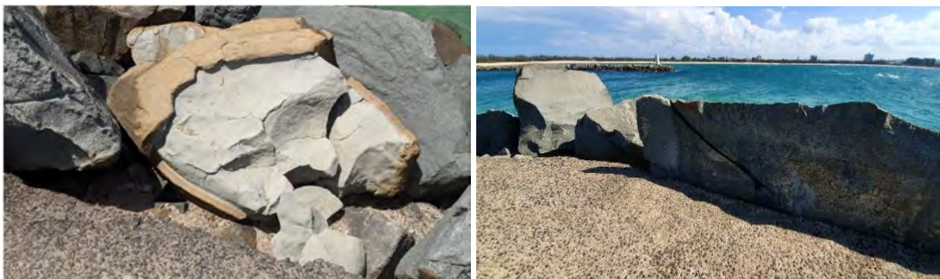
Figure 4.5 (a) weathering of the Kuluin Quarry Rock on the crest of the Mooloolaba Breakwater (seaward side) and (b) fracturing of larger rock armour (lee side)
