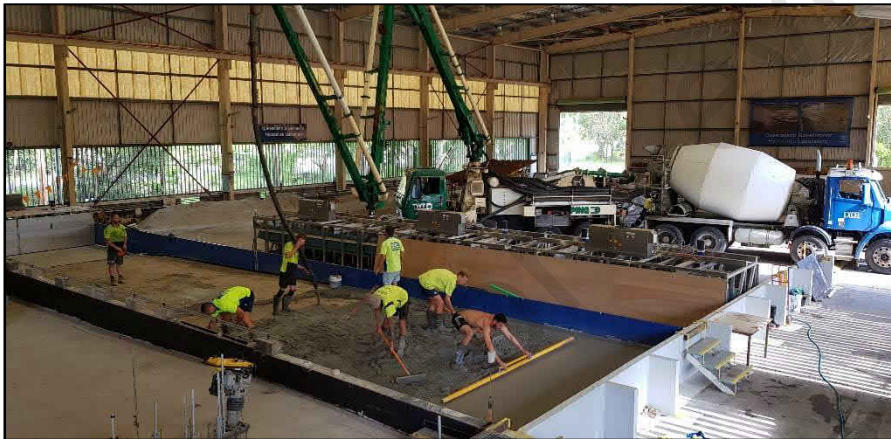
Figure 10: Flume bathymetry construction - supporting walls installation, road base fill and compaction progressing.
