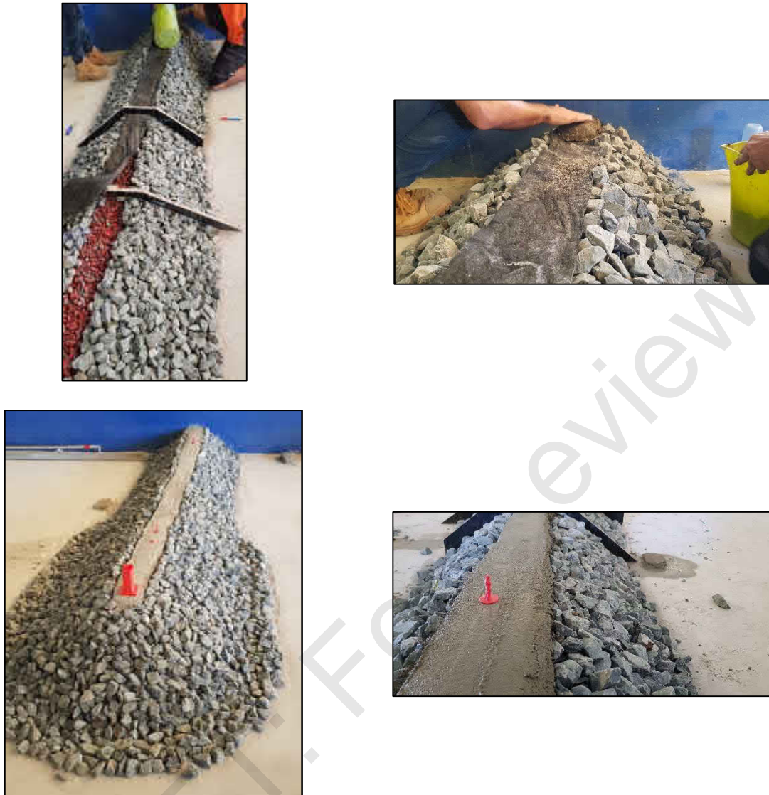
Figure 16: installation of the 5m wide walkway.
