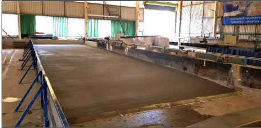
Figure 12: Completed concrete bathymetry.
