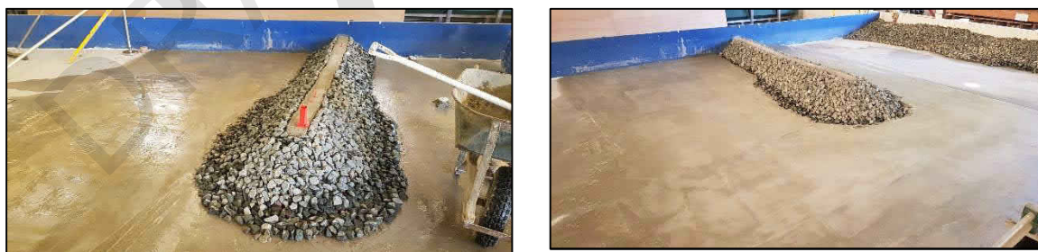
Figure 14: Installation of the removable bathymetry (weak grout) (left). Completed bathymetry (right).
