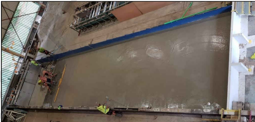
Figure 11: Concrete pour progressing.
