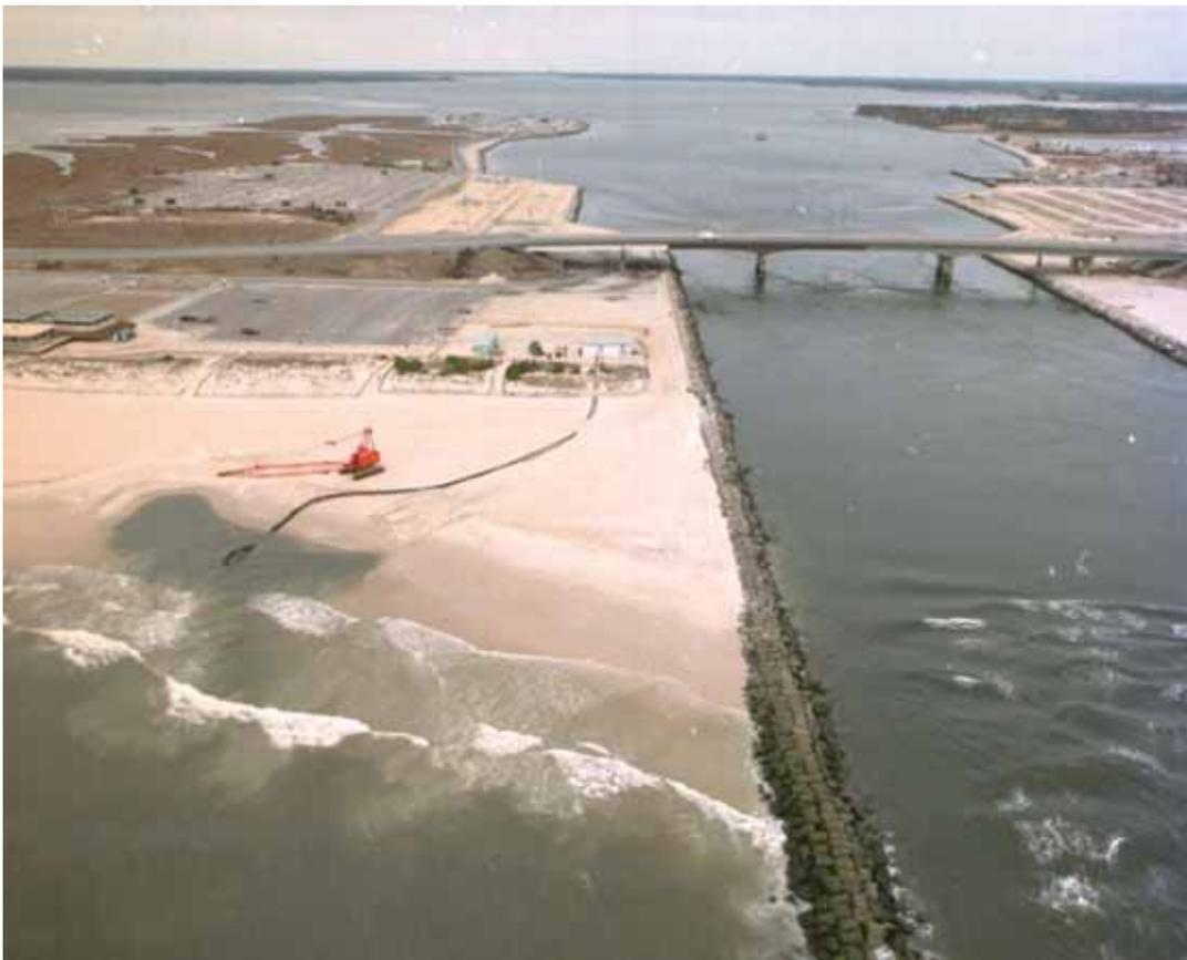
**Figure 7-7 Crane-mounted Mobile Jet Pump Sand Bypass System - Indian River Inlet, Delaware (USACE, 2013)**
