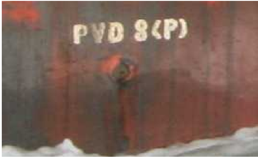
Figure 22 - Wooden Bung in Stern Discharge Outlet
