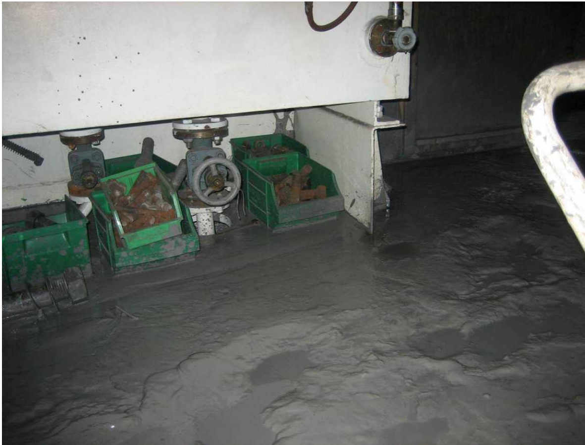
Figure 16 - Slurry on the Access Walkway to the Hot Workshop
