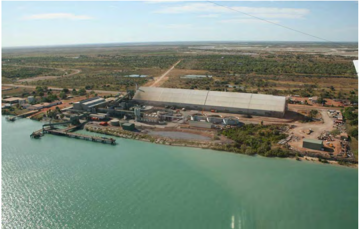
Figure 2 - The Wharf and Storage Shed
