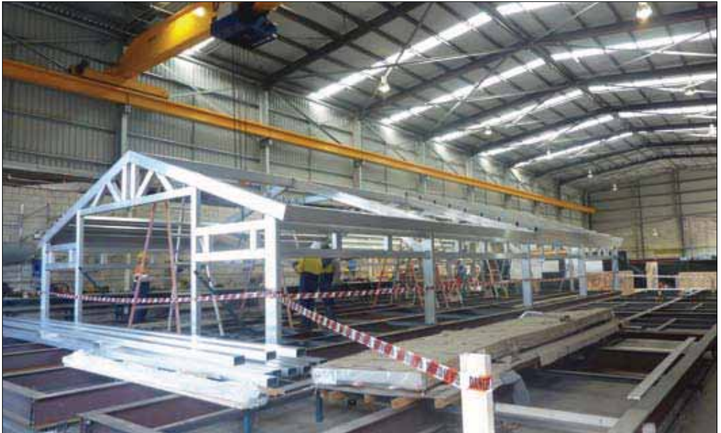
Above: Construction of roof structure.
