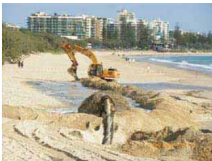
Above: Mooloolah River entrance dredging and beach nourishment.
