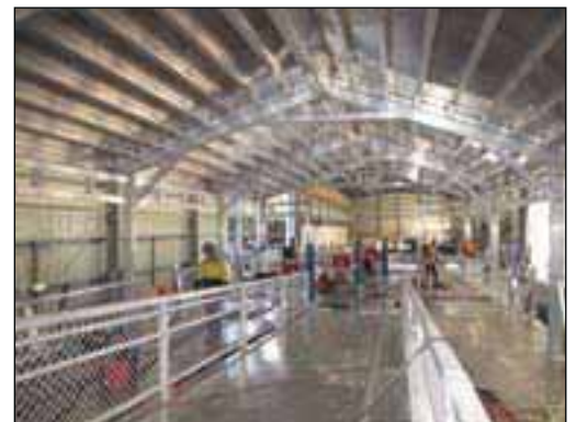
Above: Roof structure being trial fitted to pontoon.
