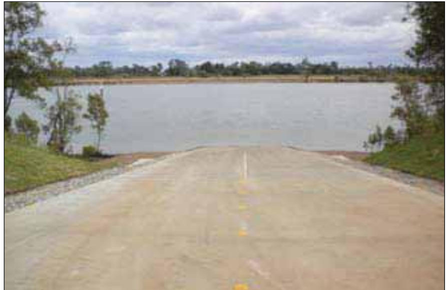
Above: New two lane boat ramp at Kalkie.
