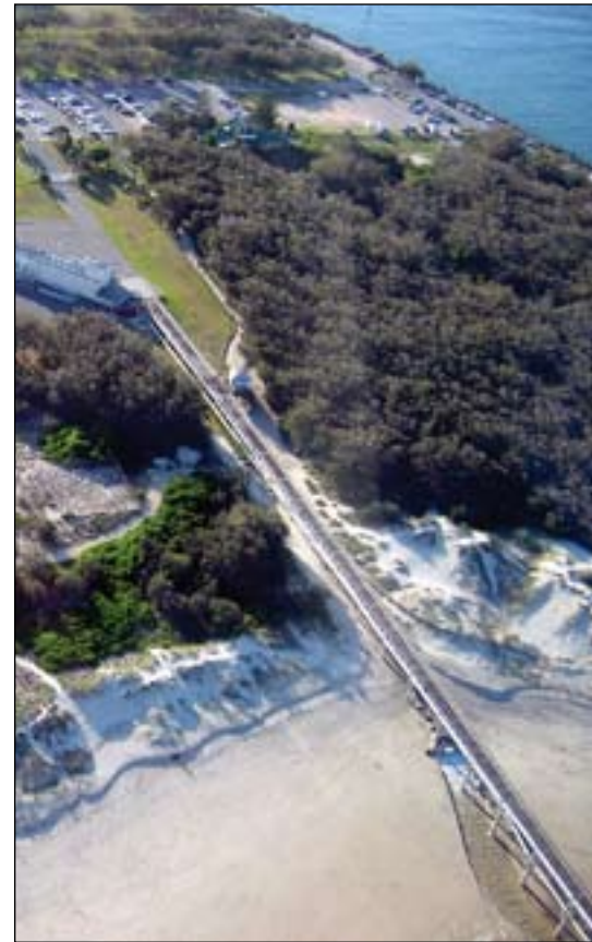
Above: An aerial view of the Sand Bypass System.
