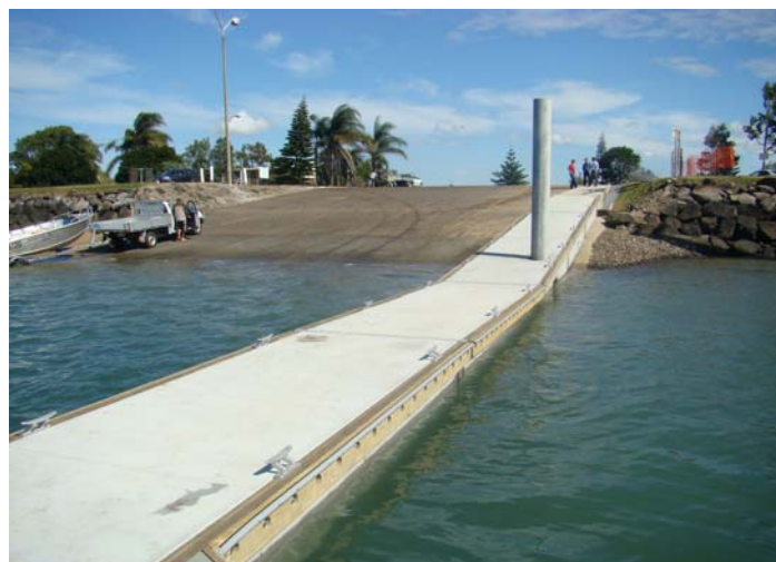
Burnett Heads Boat Harbour boat ramp & floating walkway
