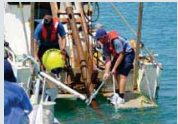
Above: crew installing the seagrass buoy mooring at Macleay Island.
