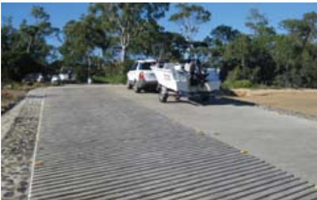
Above: New Gatakers Landing ramp, Hervey Bay.
