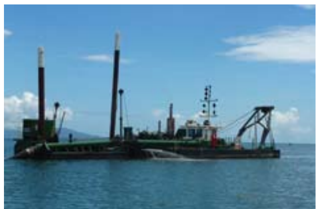
Above: Dredging works in Port Douglas in January 2010.
