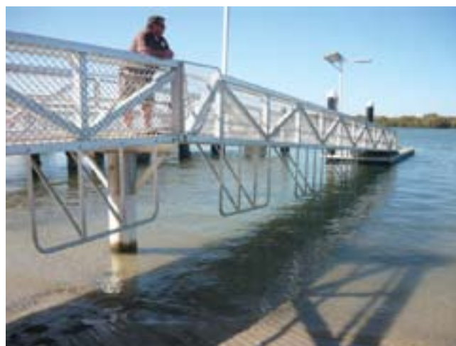
Above: New pontoon at Jacobs Well.
