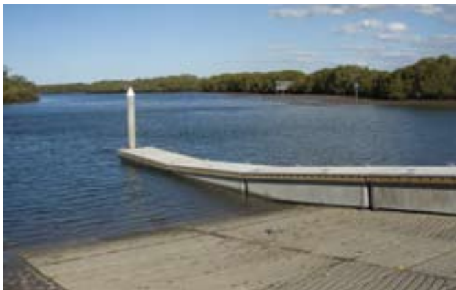
Above: Upgraded ramp and floating walkway at Sinbad Street, Shorncliffe.
