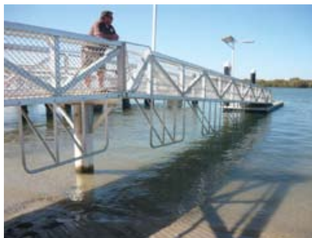
Above: New pontoon at Jacobs Well.
