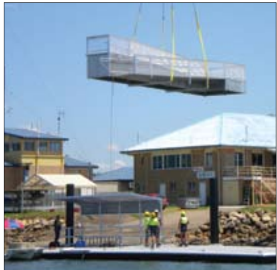
Right: Manly Boat Harbour, community sports pontoon during construction.
