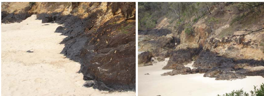
Figure 27: Oiled rocks and cliffs at Honeymoon Bay – trial cleaning with high-pressure water jets (Moreton Is. North Coast 18/3/09).
