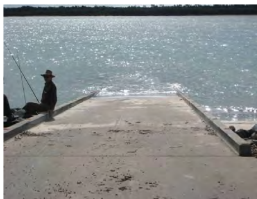
Ross Street boat ramp – single lane
