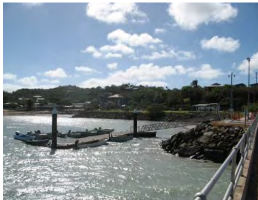
Existing pontoon at Thursday Island
