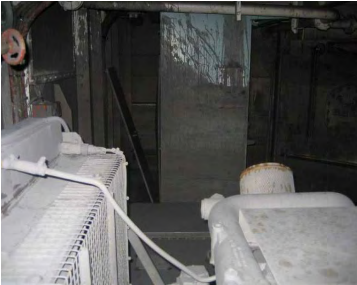
Figure 6 - Inside the Emergency Generator Room
