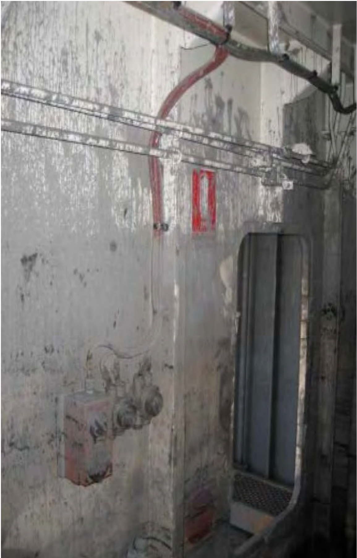
Figure 5 - The Hot Workshop Depicting Slurry Marks
