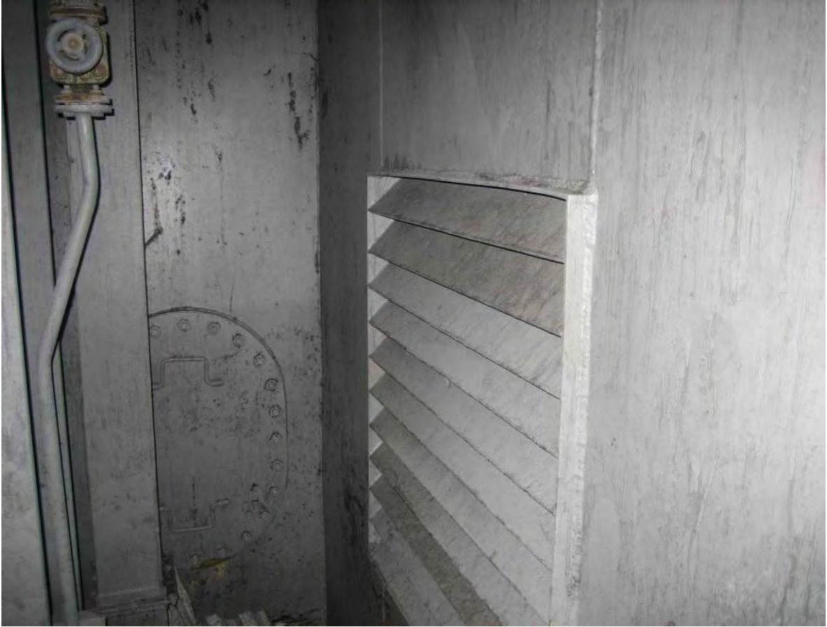
Figure 14 - Louvered Vent from the Emergency Generator Room
