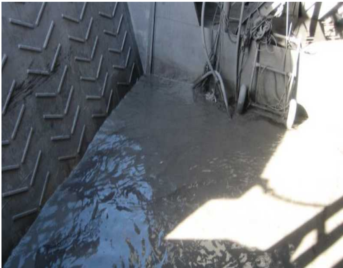
Figure 4 - Water in the Aft Well Deck
