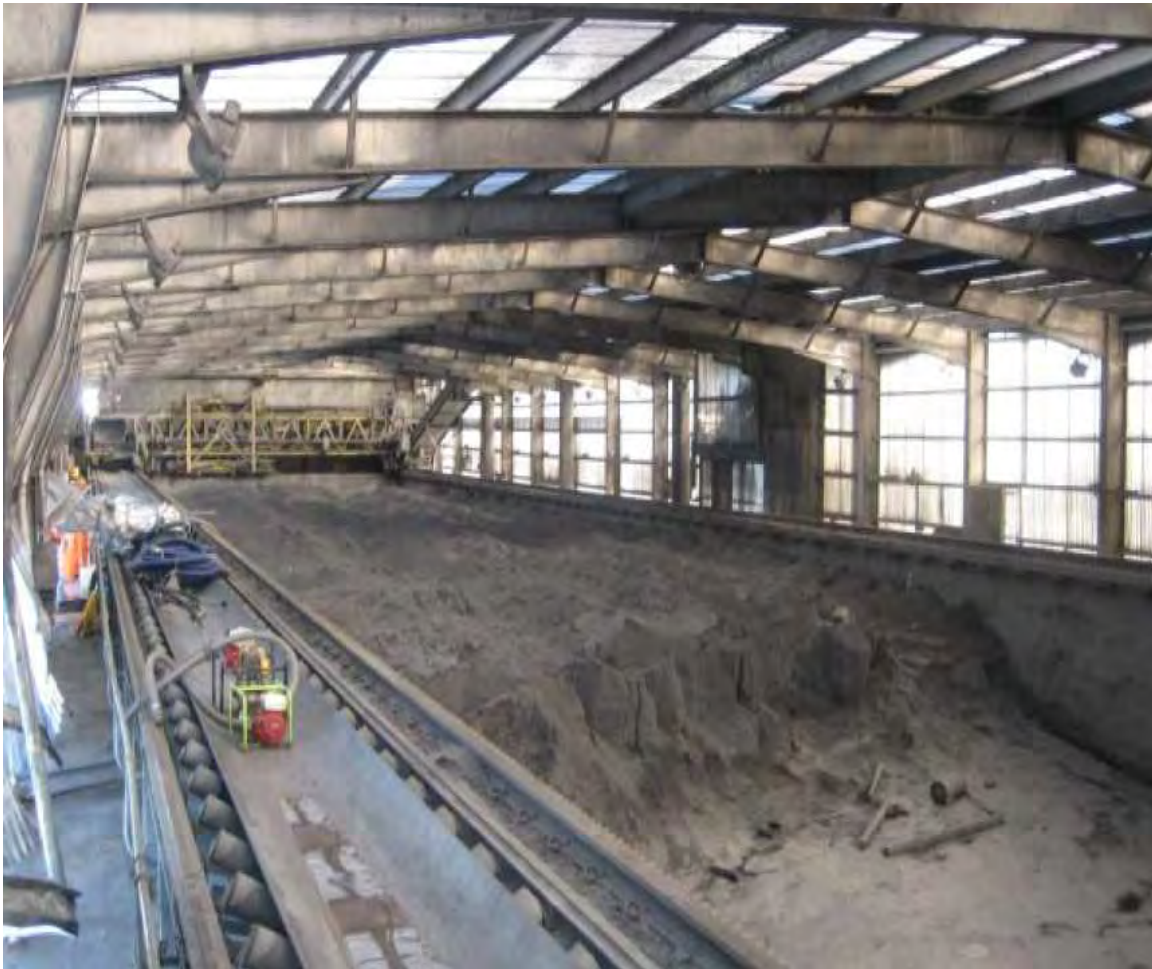
Figure 10 - Debris in the Cargo Hold
