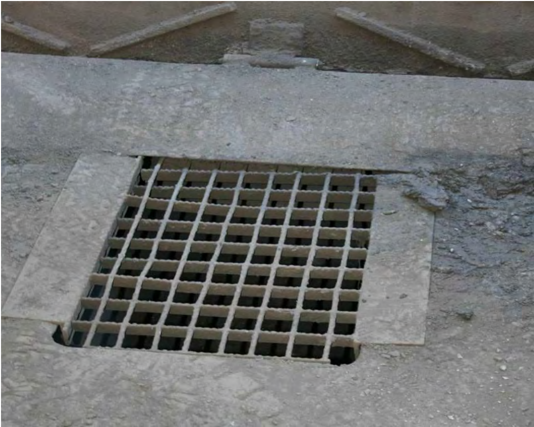
Figure 5 - The Aft Well Deck Sump
