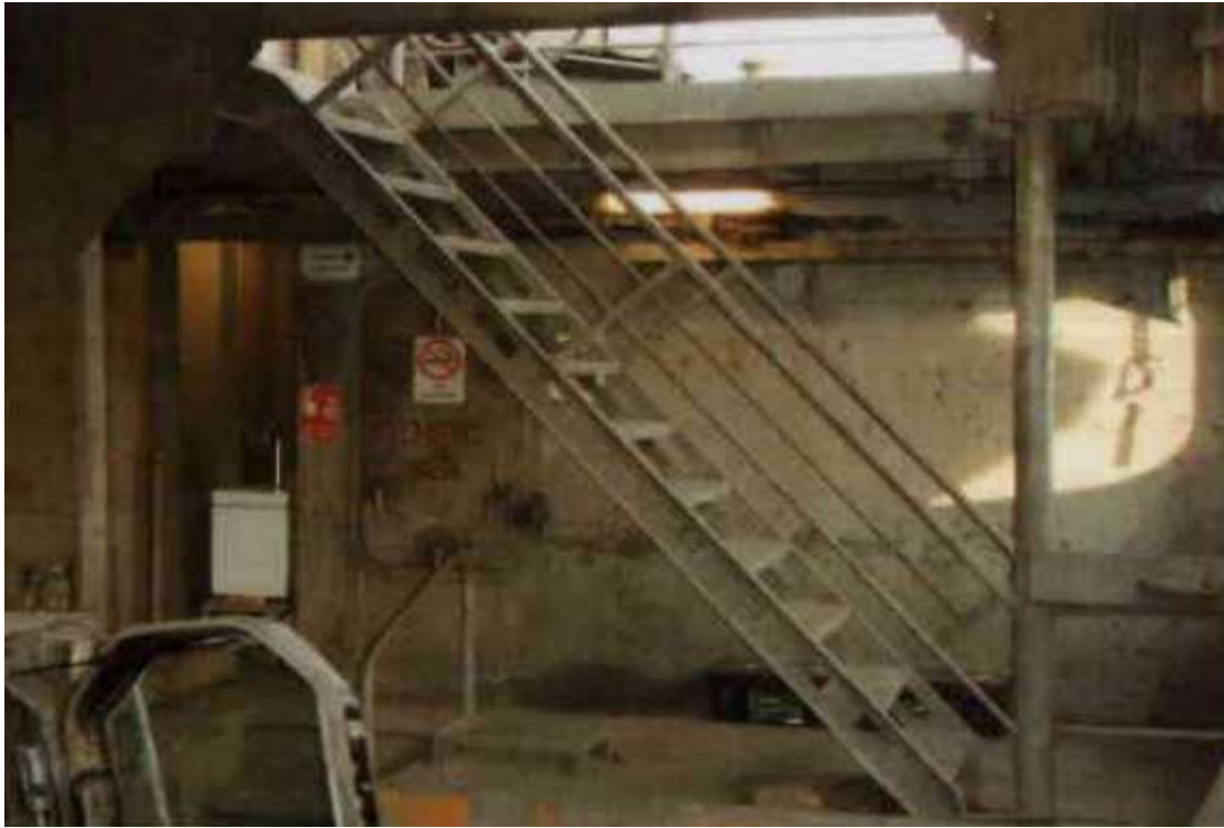
Figure 7- The Emergency Generator Room
