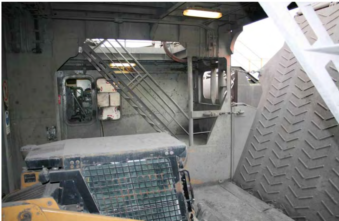
Figure 2 - The Aft Well Deck and Emergency Generator Room
