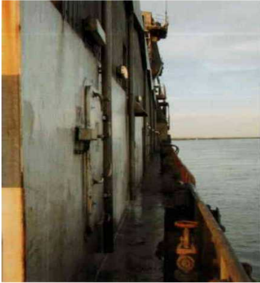
Figure 3 - Starboard Deck and Downpipes
