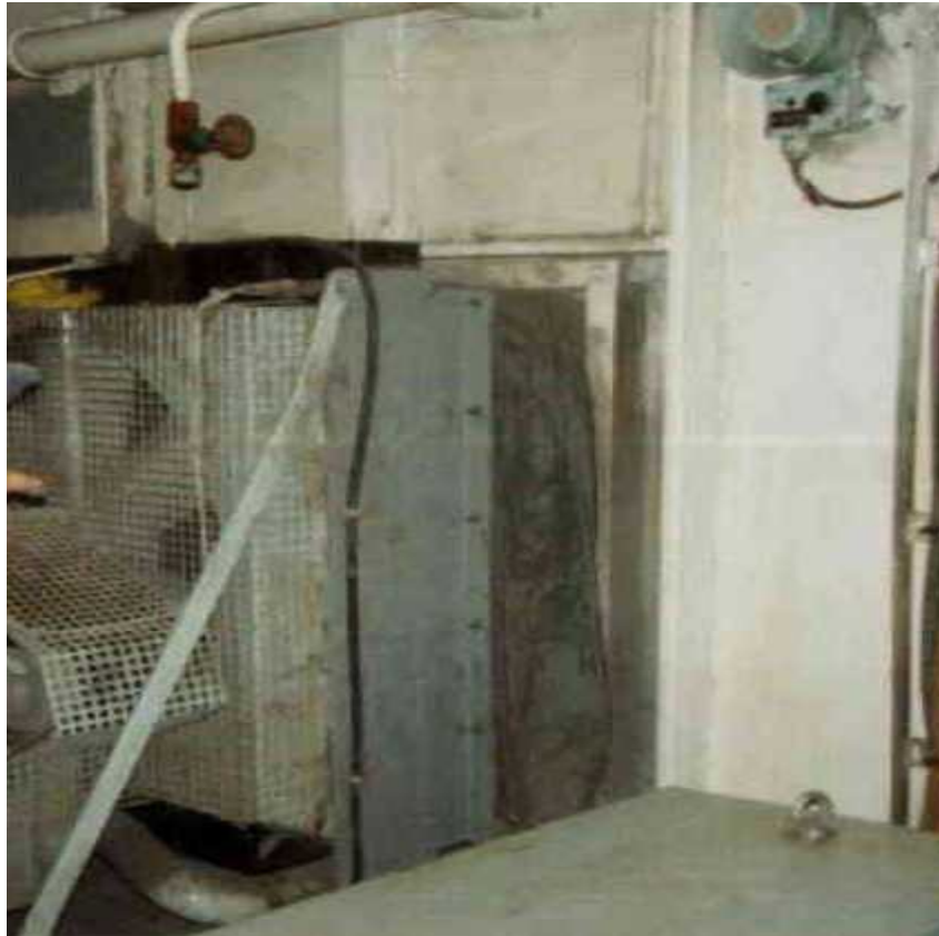
Figure 9 - Emergency Generator Radiator adjacent to Vent
