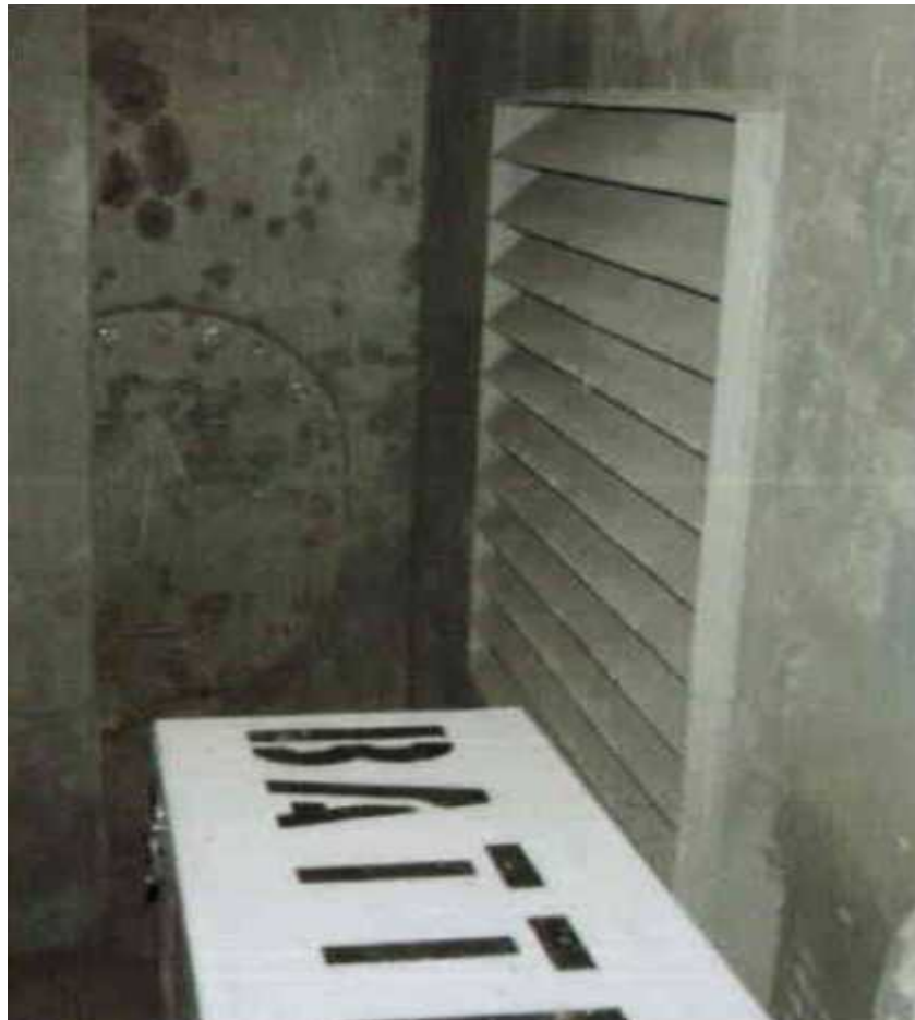
Figure 8 - Radiator Vent - Emergency Generator Room
