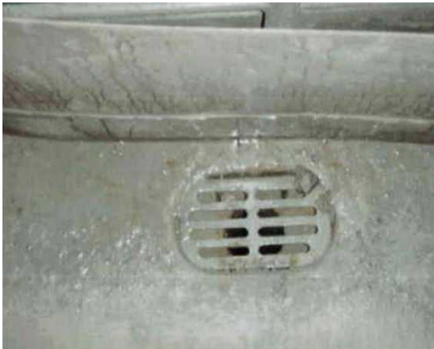
Figure 4 - Deck Drain on Starboard Walkway
