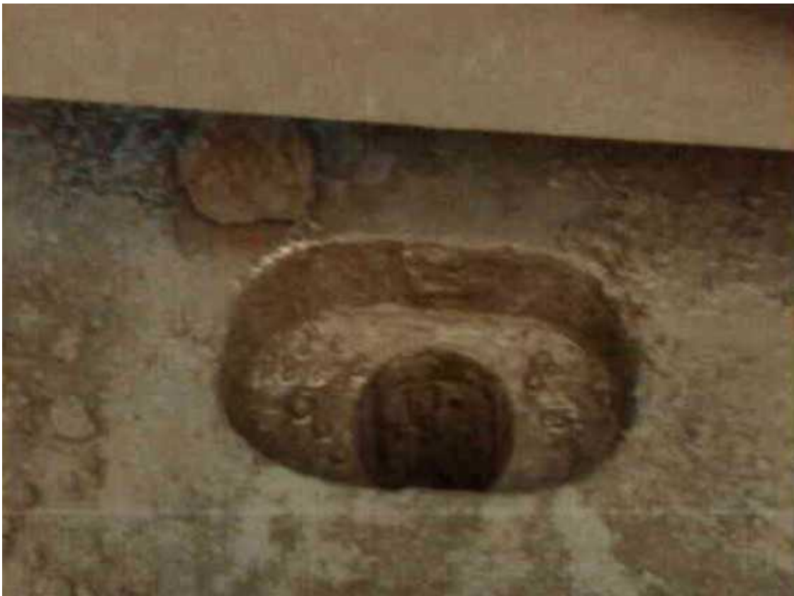
Figure 6 - Deck Drain on the Port Side Walkway
