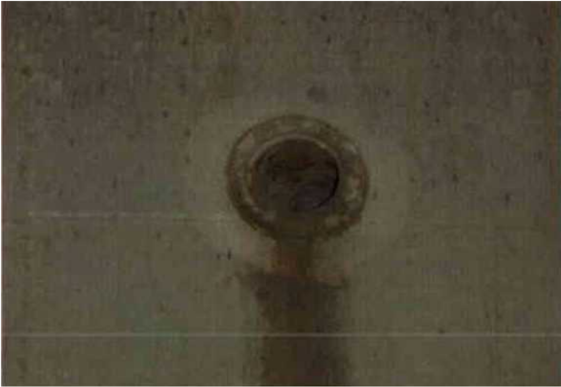
Figure 9 – Blocked Washdown Ports under the Conveyor
