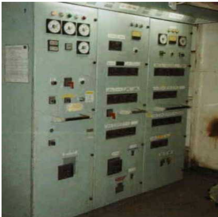
Figure 10 - Emergency Generator Switchboard
