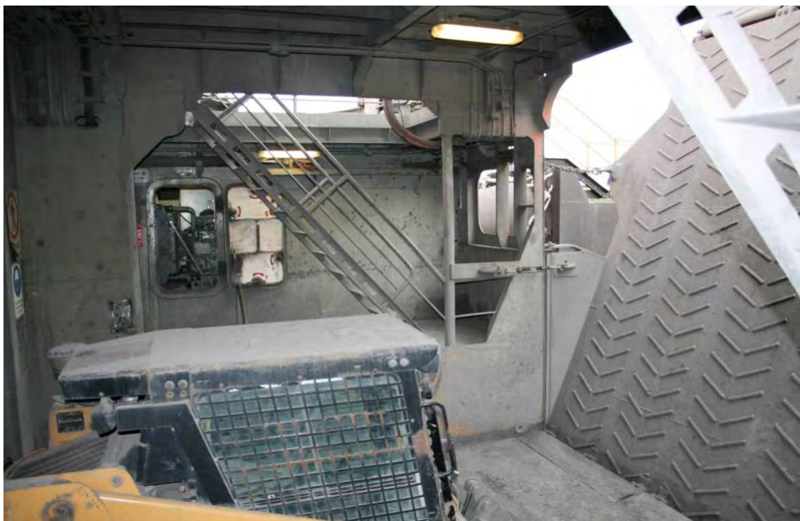
Figure 2 - The Aft Well Deck and Emergency Generator Room
