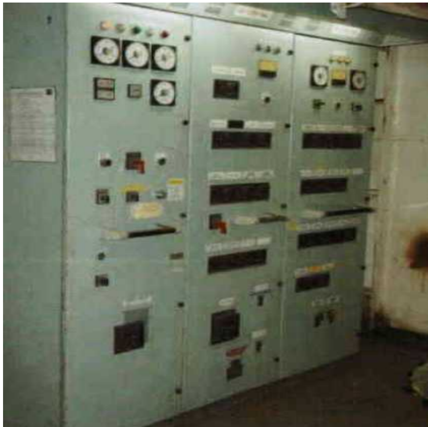
Figure 10 - Emergency Generator Switchboard
