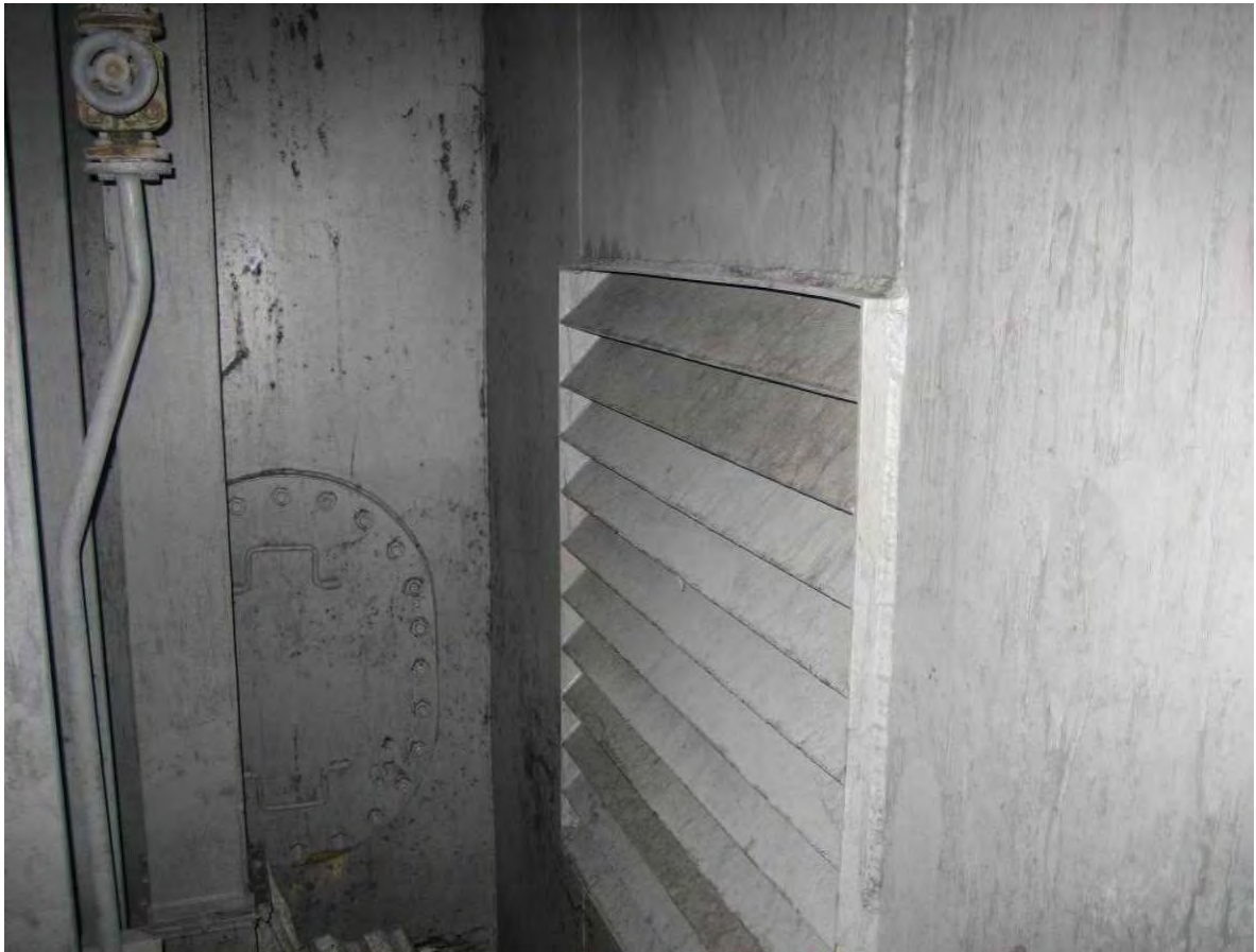
Figure 14 - Louvered Vent from the Emergency Generator Room
