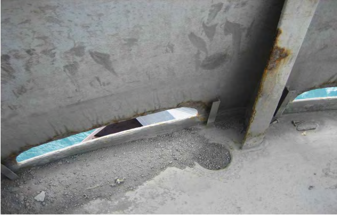
Figure 20 - Freeing Ports - Starboard Aft Quarter Deck
