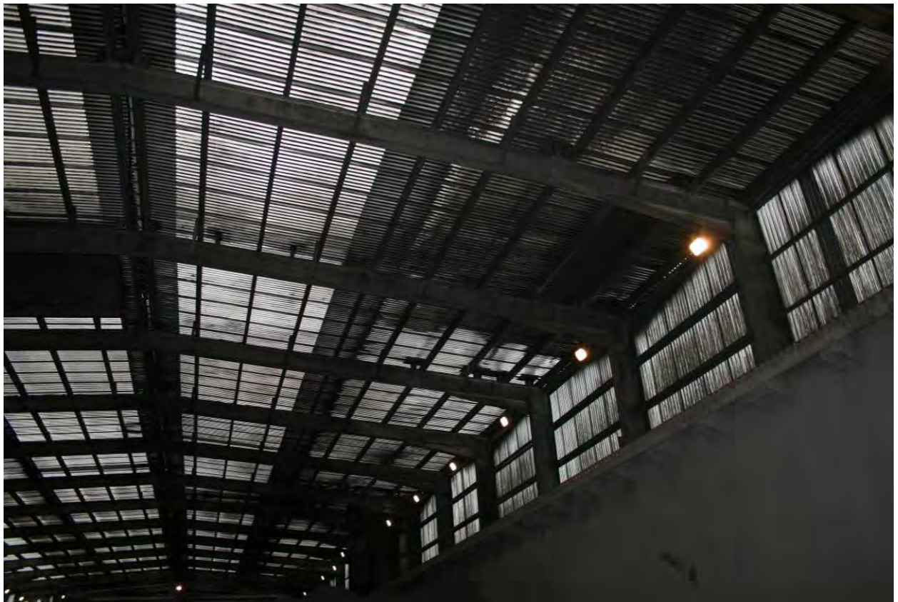
Figure 4 - The Canopy Roof
