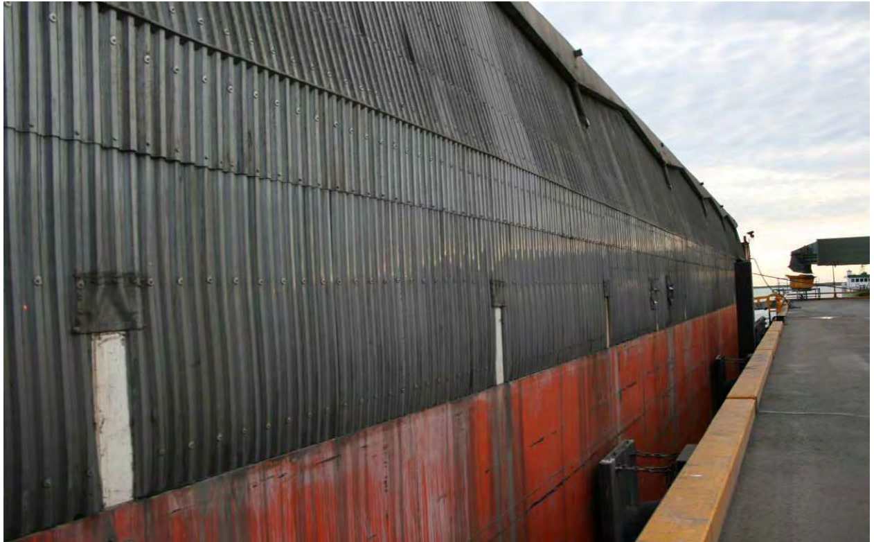
Figure 10 - Side of the Canopy
