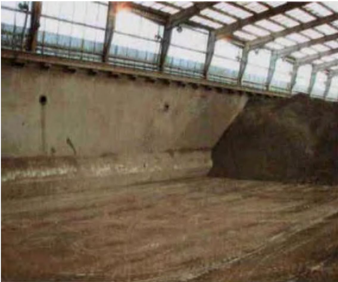
Figure 8 - Washdown Outlets from under the Conveyor
