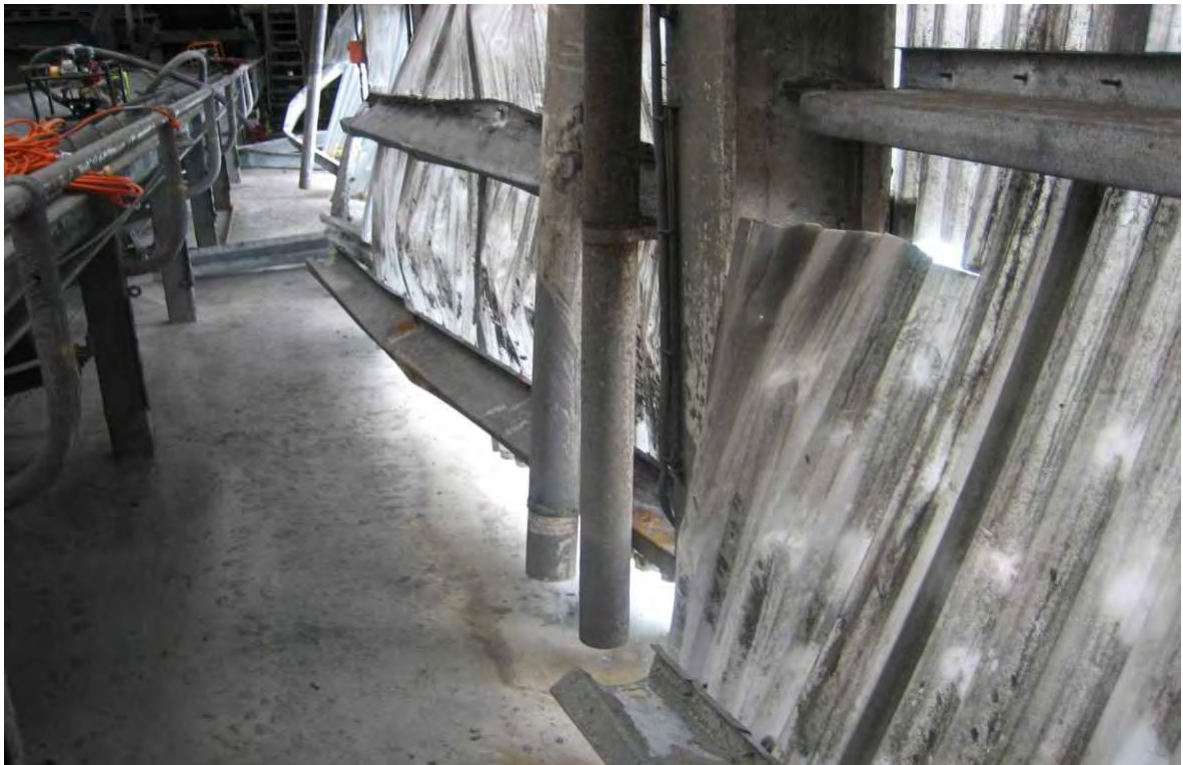
Figure 15 – Damage and Down Pipes and to the Port Side Deck
