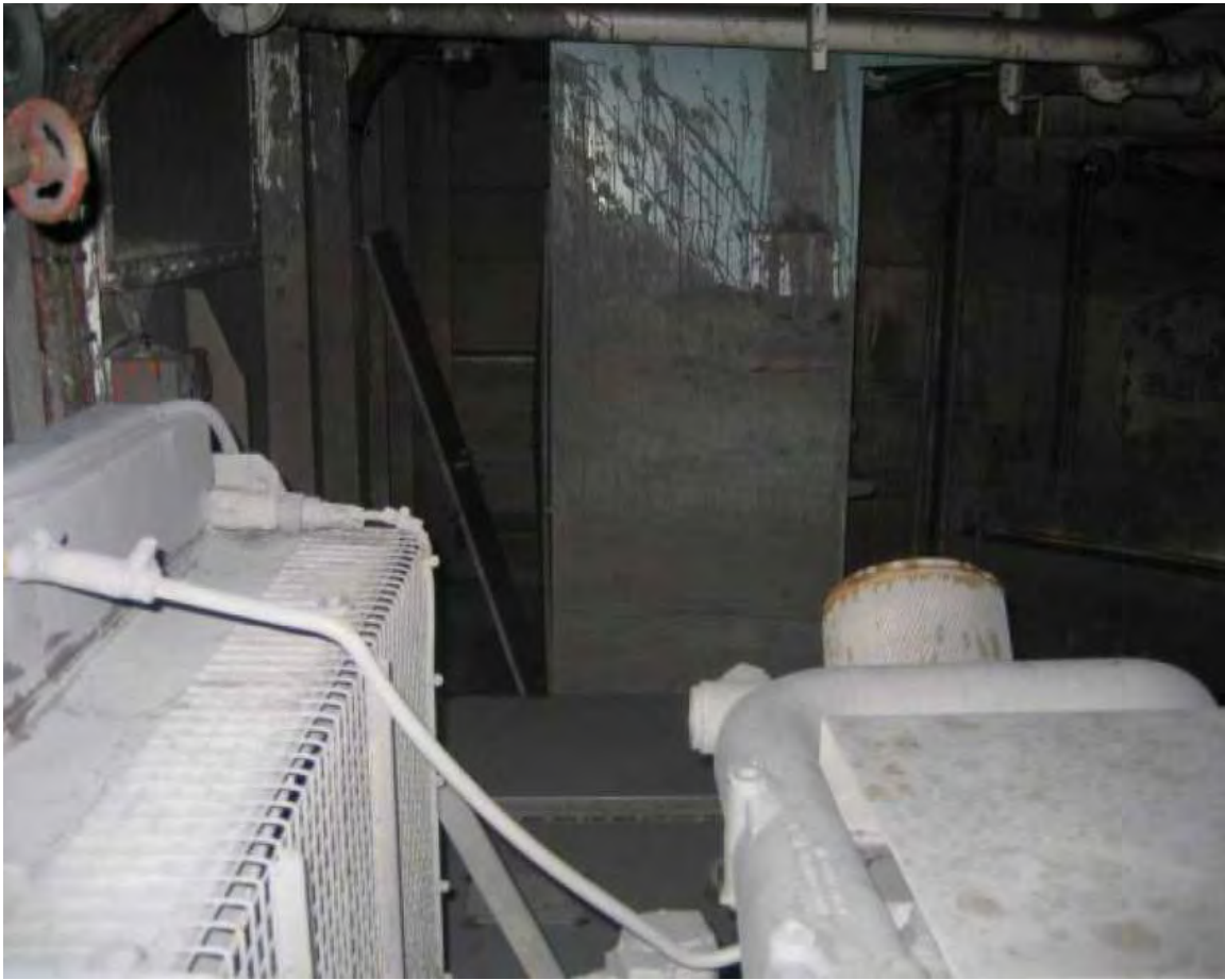
Figure 6 - Inside the Emergency Generator Room
