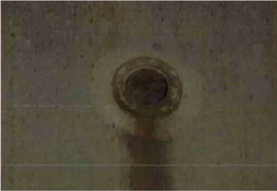
Figure 9 – Blocked Washdown Ports under the Conveyor
