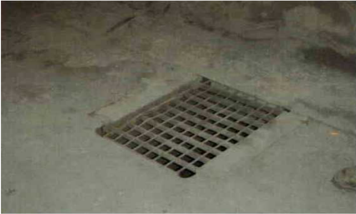
Figure 7 - Aft Well Deck Sump
