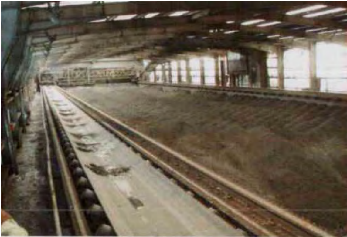
Figure 10 - Conveyor Port Side Walkway Showing Concentrate Deposits on Port Deck
