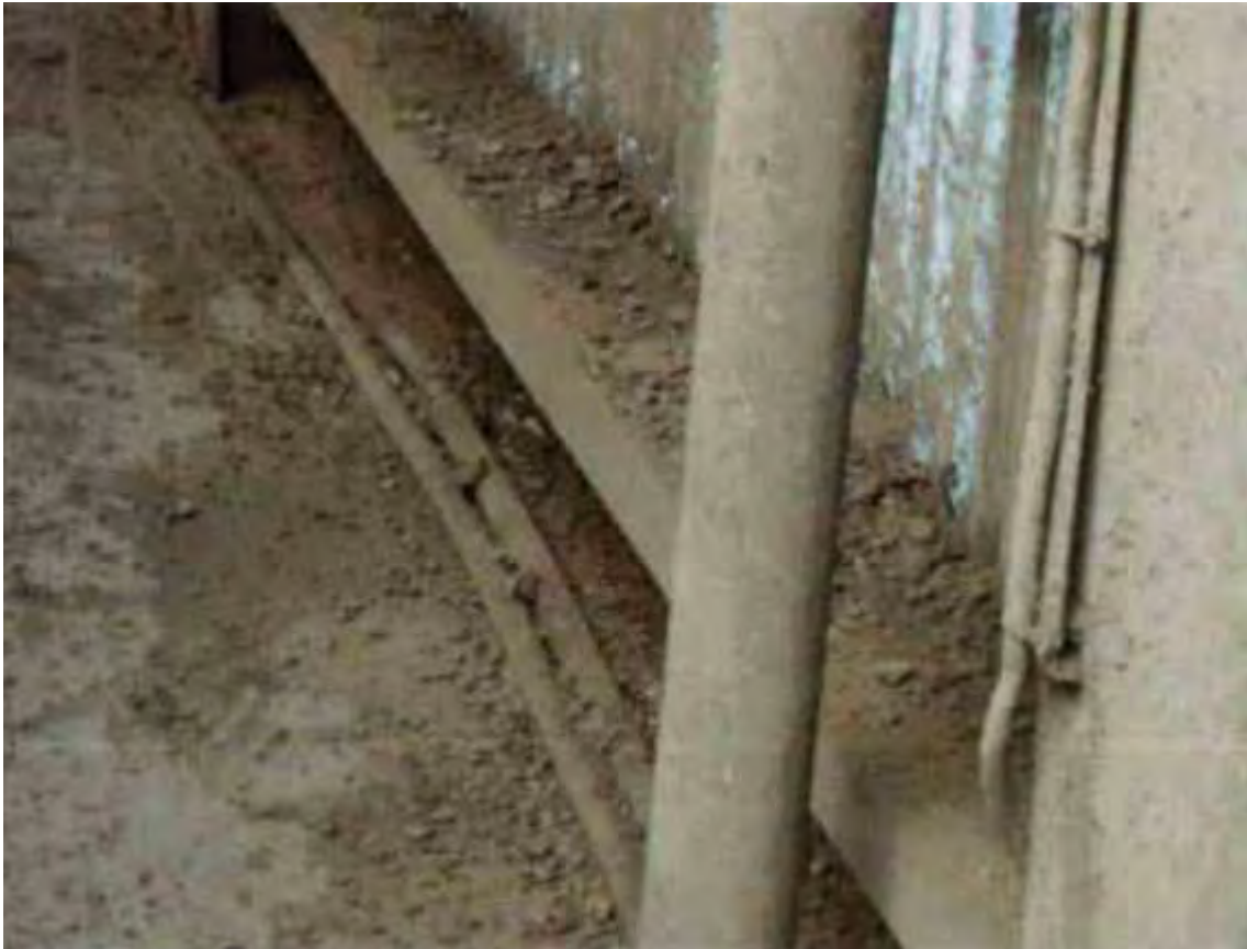
Figure 5 – Downpipe Extending from Roof Gutter on the Port Side Walkway
