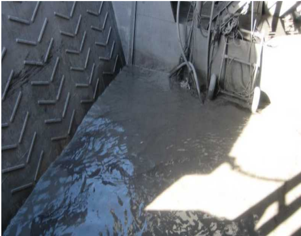
Figure 4 - Water in the Aft Well Deck
