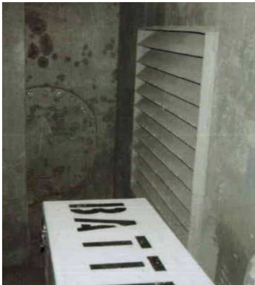
Figure 8 - Radiator Vent - Emergency Generator Room
