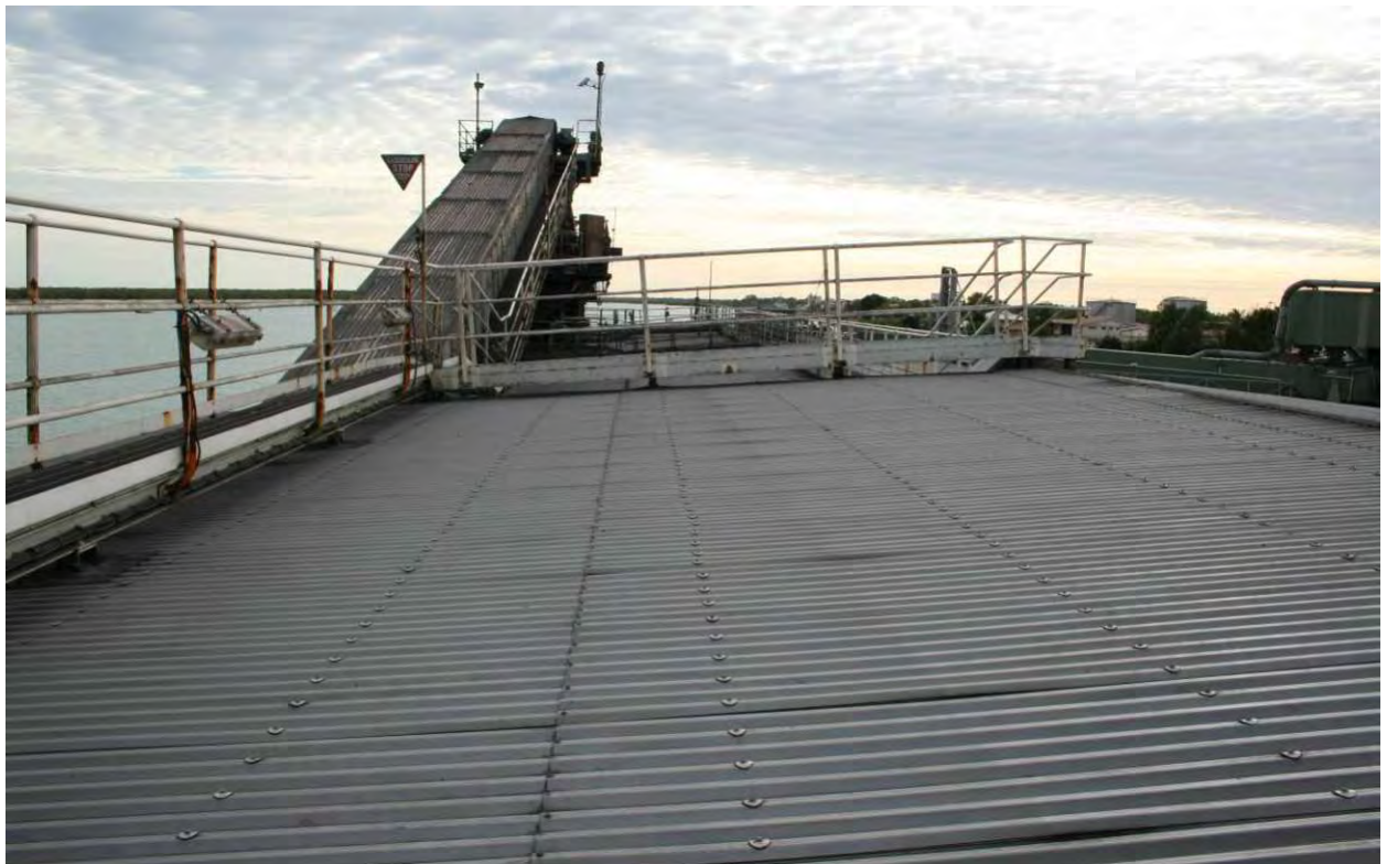
Figure 9 - The Canopy Roof
