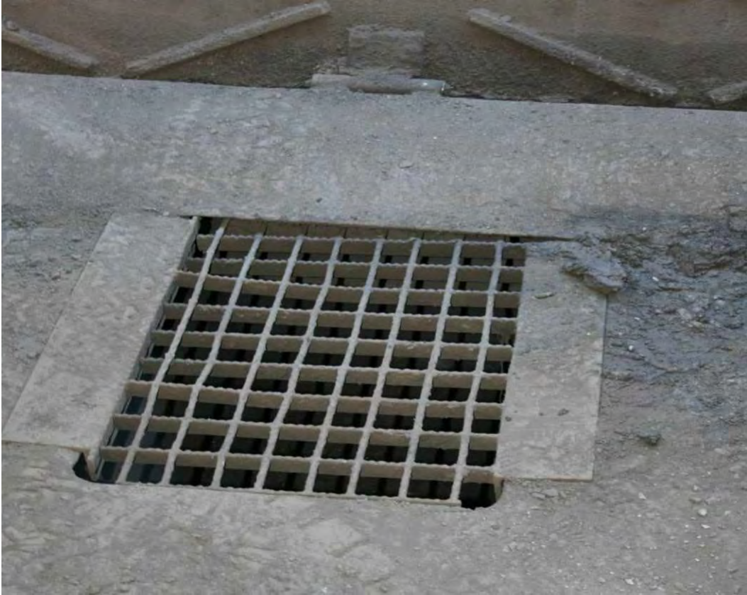
Figure 5 - The Aft Well Deck Sump
